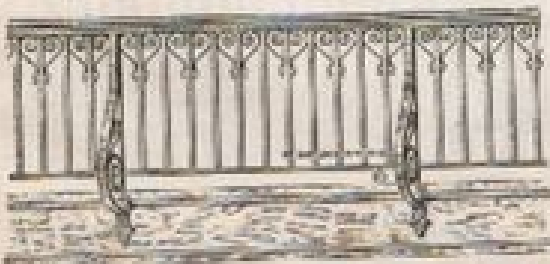
No. 87—Gallery or Mezzanine Railing
